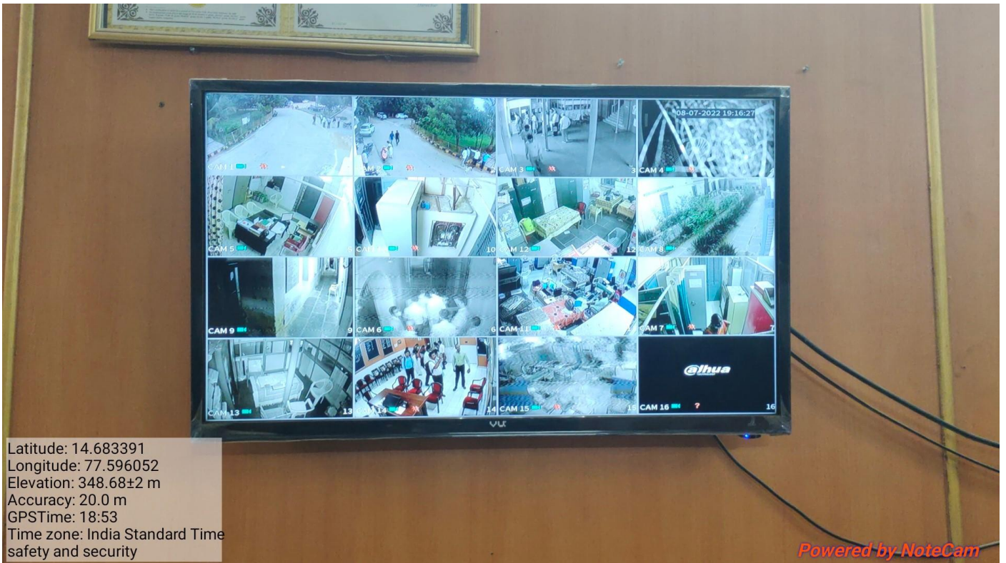
CC Cams controlling Unit in the Principal Chamber
